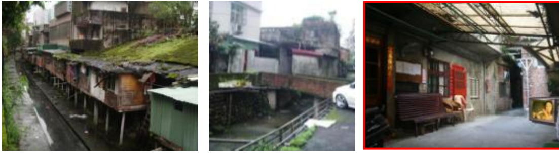
Fig.6~8 Liugongjun Waterway (bottom) and community (up), small route cross the community which called informal MDV.
