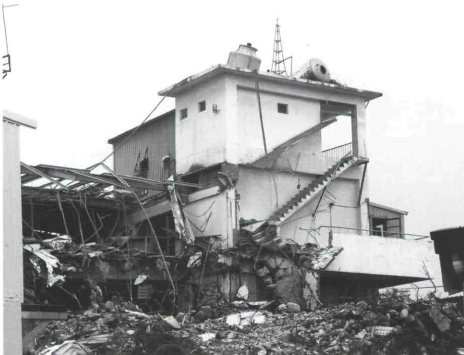
Figure 16. Buildings destroyed in the Chi Chi Earthquake in the city of Pouli. 2001.
